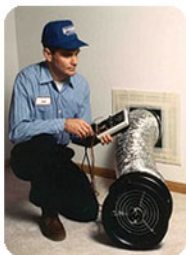
HERS rater pressure testing a duct system
